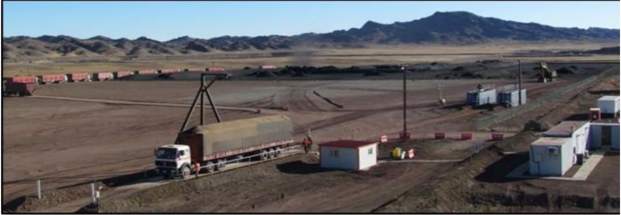
The CBY at BNU Mine
