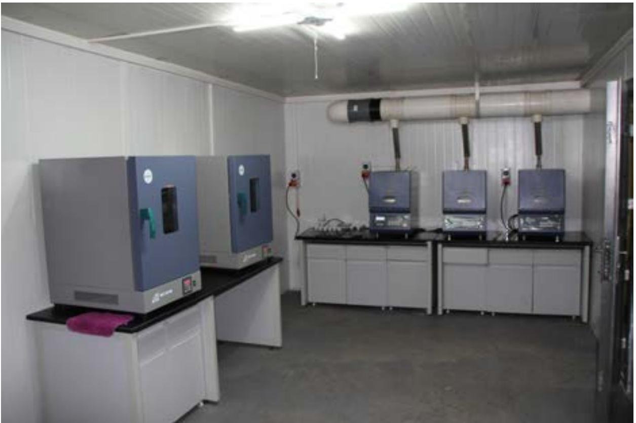
Below: Laboratory construction on site now complete.
